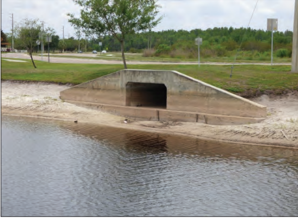
Stormwater Drainage Box Culvert
