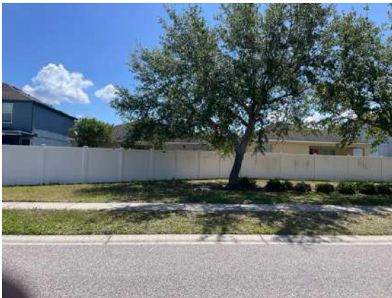
Observation Assigned To Maintenance Crew Be sure to lift any water weighed branches back to 10 feet. Continue to do so.
