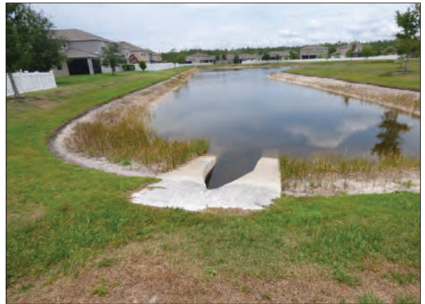
Stormwater Drainage Mitered End Section
